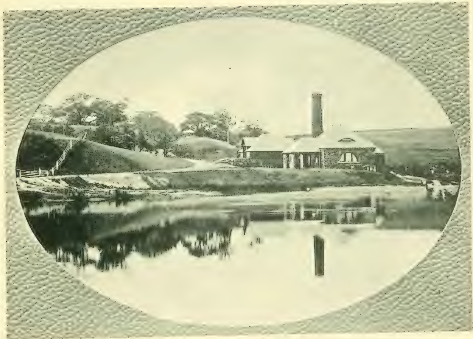
PUMPING STATION—COTTAGE CITY.
